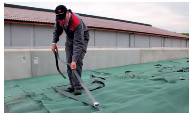
Step 4: Sheets are then tensioned with belts and ratchets.
