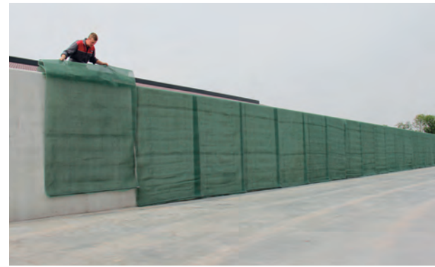
Step 1: Woven sheets are laid out with a 25 cm overlap on either side of silage pit.
