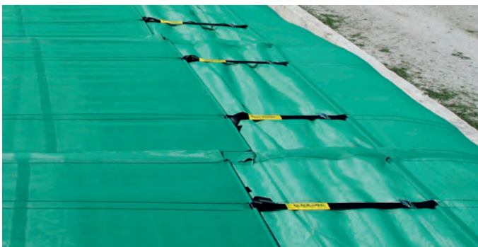
New cover system – rapidly installed
